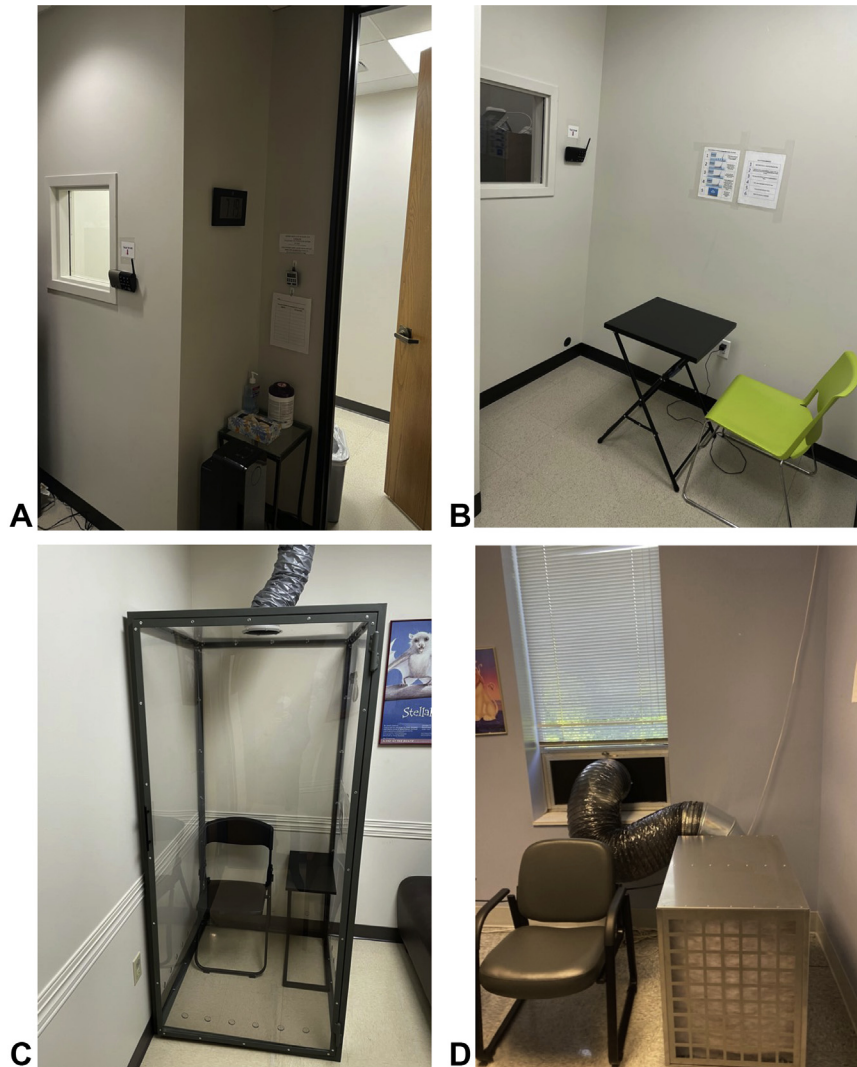
FIGURE 3. Pulmonary procedure room modifications. (A) Pulmonary procedure room with anteroom allowing visual and intercom communication between the staff and patient with high-flow exhaust (exterior). (B) Pulmonary procedure room with anteroom allowing visual and intercom communication between the staff and patient with high-flow exhaust (interior). (C) Pulmonary procedure Plexiglas chamber in the examination room with high-flow exhaust. (D) Pulmonary procedure examination room with high-flow exhaust.
